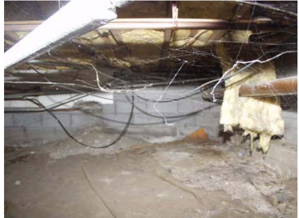
Parish center crawl space.
