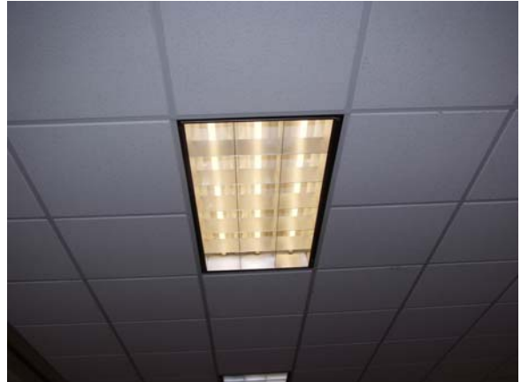
18 cell parabolic lighting fixture, typical of office lighting a few years ago.
