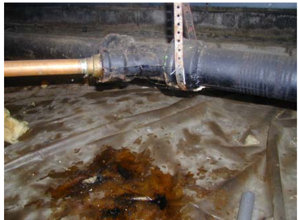
Leaking joint.
