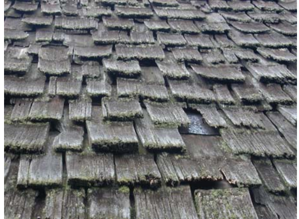
Closeup of church cedar shakes.
